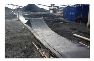
back on itself to form the flaked piles. As a minimum we recommend that the diameter of any pipe sections used be the same as the diameter of the core section of the spool the belt was delivered on. Careful thought also needs to be given to how the flaking will affect roll sequencing given that all rolls are delivered with the assumption that they are all installed in the direction of travel. Smartwire and sensor loop location may also have to be considered at this stage.
