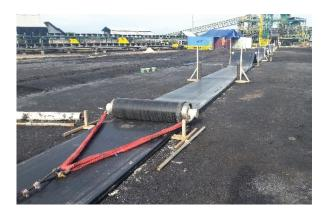
Careful consideration needs to be given to the condition of the working floor area where the belt will be flaked, the length and height of the flaked piles, the method and equipment used to move the belt as it is uncoiled and flaked, the equipment used to make-safe and secure the piles so that belt is not unstable and the angle of wrap as the belt is folded
